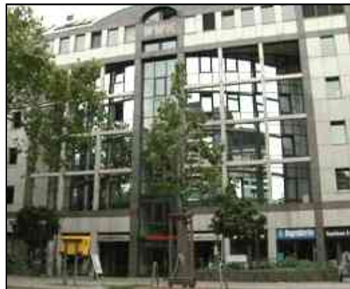
Photo of the building at Hardenbergstr. 8 in Berlin. The company occupies two floors in the upper part of the building including a technical zone with electro-static-damage (ESD) protected work areas.
