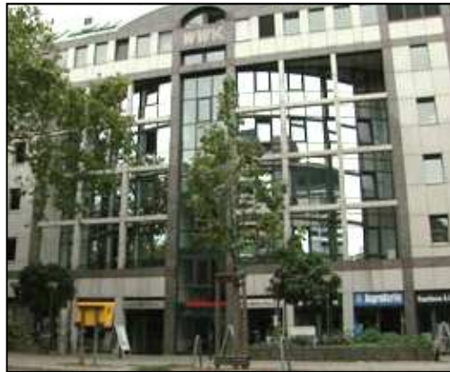
Photo of the building at Hardenbergstr. 8 in Berlin. The company occupies two floors in the upper part of the building including a technical zone with electro-static-damage (ESD) protected work areas.
